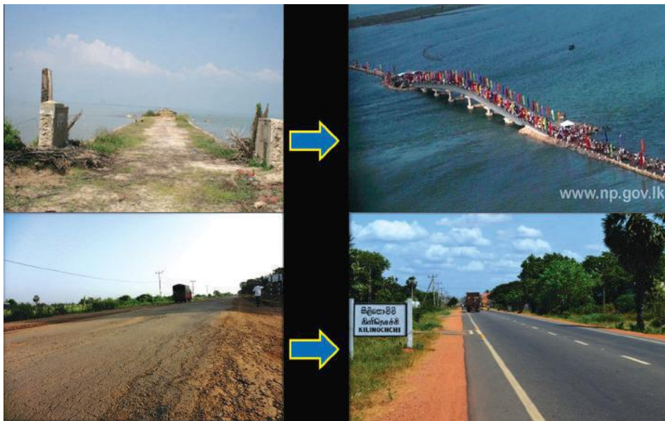
Sangupiddy Bridge connecting Poonarin to Jaffna (288 m) was built at a cost of Rs. 1.037 billion and 153 km of road were constructed to extend the A9 Highway from Anuradhapura-Galkulama to Jaffna at a cost of Rs. 19,125 million (images from Northern Provincial Council website: http://www.np.gov.lk/ ).
